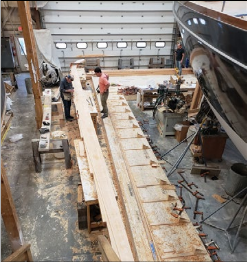
This is the keel for the 55-foot Wheeler that will be built this winter at Brooklin Boat Yard in Brooklin. When taking this photograph, I was informed there are now two of these on order so they will be making double of everything
