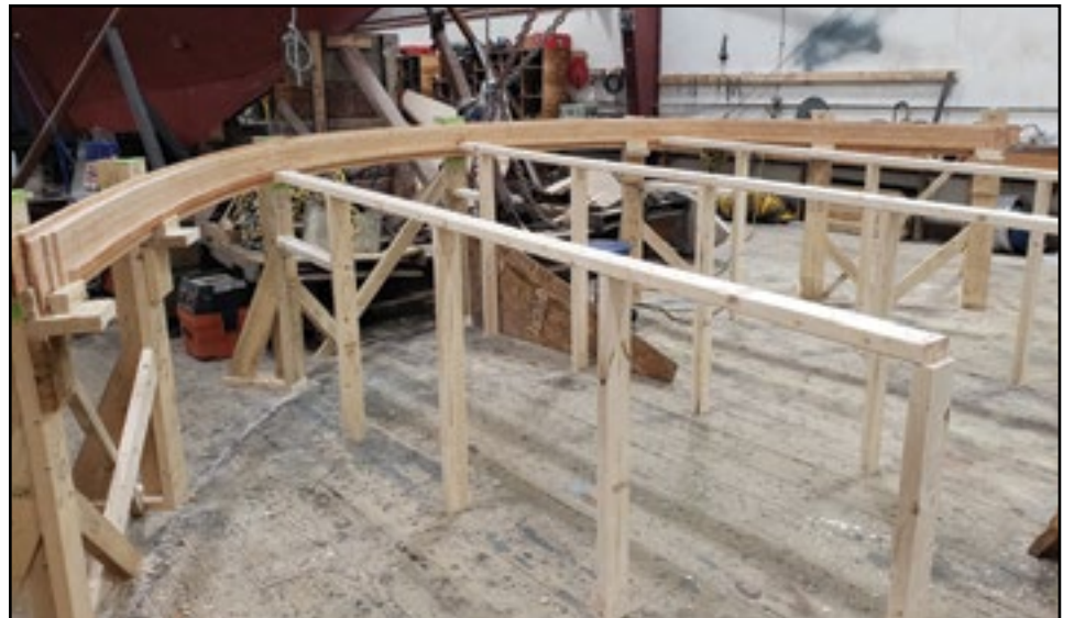
The Shipyard at Boothbay Harbor, Bristol Marine is in the process of replacing the stern deck on KATAHDIN up on Moosehead Lake. They took all the measurements and incorporated a twist into their jig, which she has, so they could build it at their shop in Boothbay.
