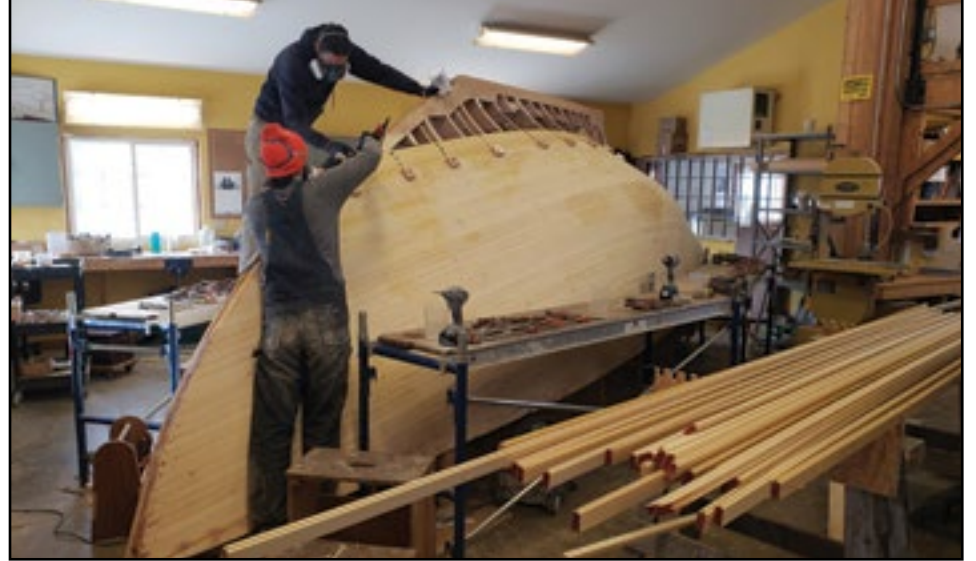
This is a 21-foot offshore cruiser, designed by Tom McNaughton of Eastport, under construction at Artisan Boat Works in Rockland. She is designed to carry one person around the globe. She has no engine, no thru-hulls and an unstayed carbon junk rig.
