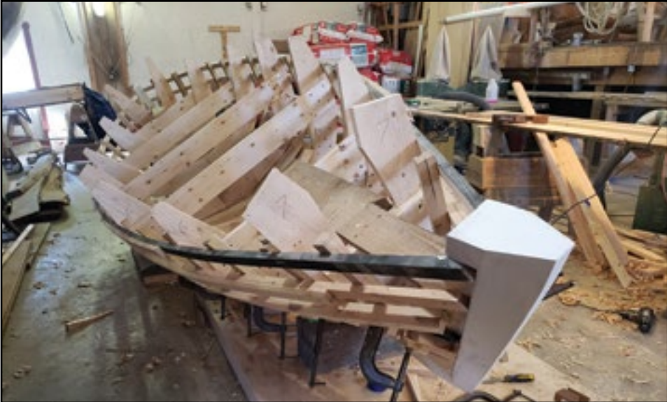
At Buxton Boats in Sunset Peter has all the molds and ribbands in place so he can start planking this Cayman catboat for a customer from the Cayman Islands in the Caribbean.
