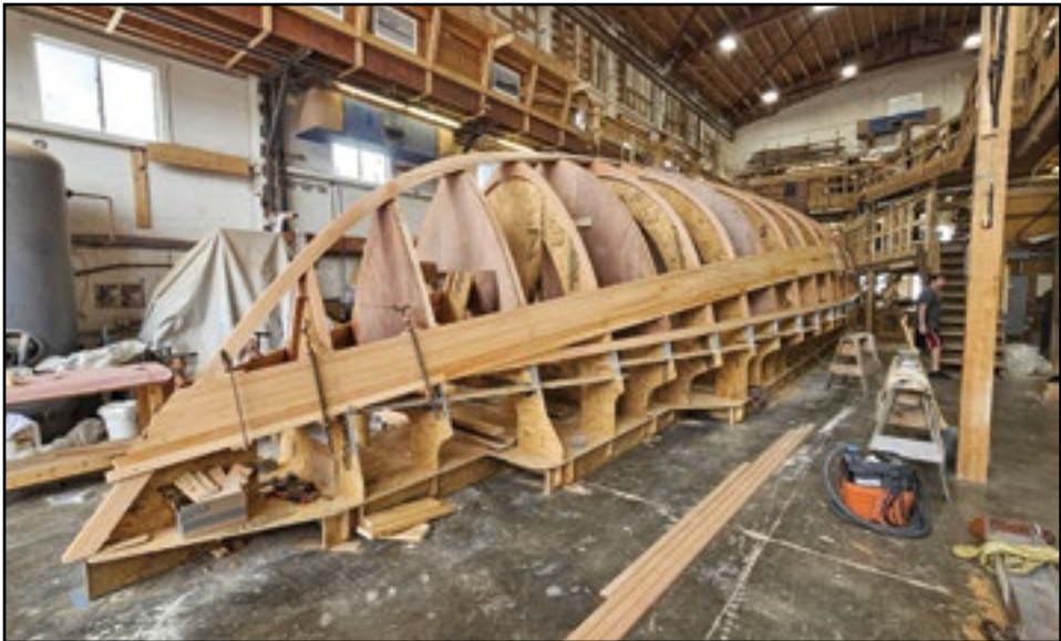
The 56-foot sailboat just starting to have her cold moulded hull formed at Brooklin Boat Yard in Brooklin.
