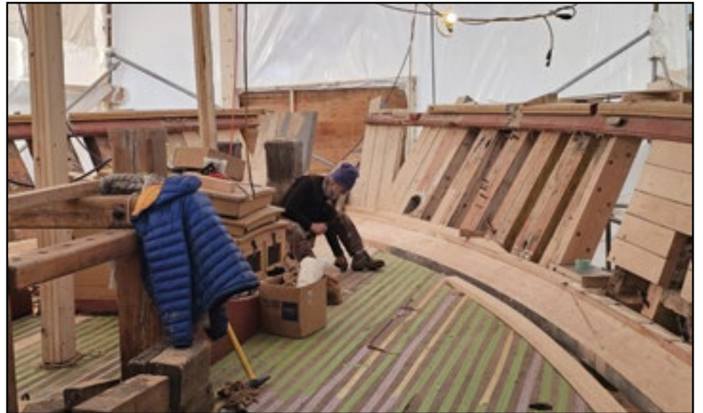
This is a view of the bow on NIAGARA, which undergoing some major repair work. Photo by: Capt. Gregory Bailey
