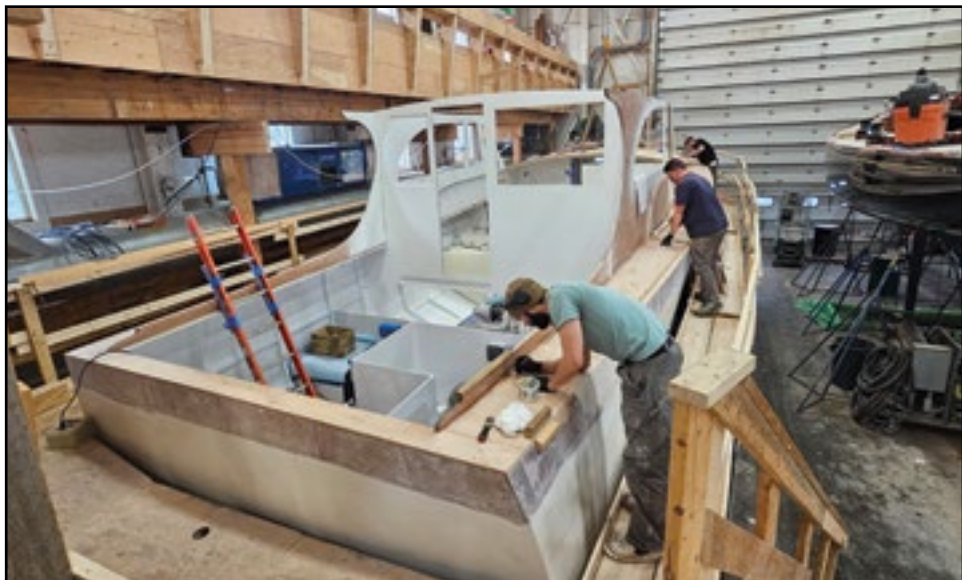
The 47 Downeast Cruiser designed by Will Sturdy and under construction at Brooklin Boat Yard in Brooklin is moving right along. The deck is down and the sides of the cabin are in.
