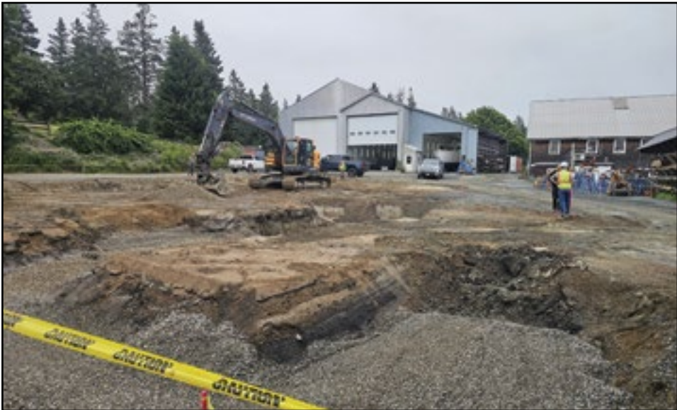
The storage building that was next to the main shop at Brooklin Boat Yard has been removed and will be replaced with a multi-bay work shop.
